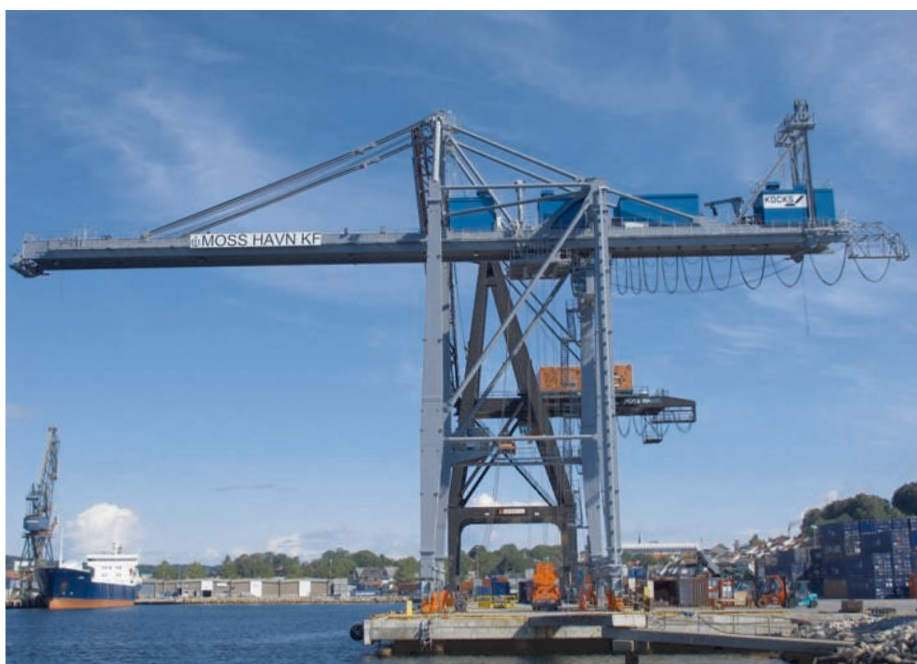
↑ Feeder Server in a Scandinavian container terminal
