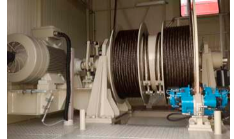
↑ Boom hoist gear
